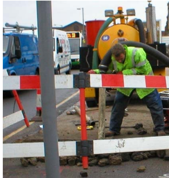
Vacuum Excavation techniques assist in trial holing for utility tracing with minimum disruption to the ground surface and the continuation of everyday life. (Picture courtesy of U Mole Ltd.)
