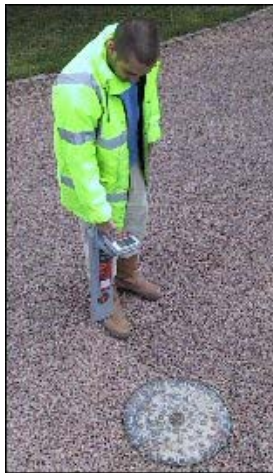
Using an EM system to trace buried services. Picture courtesy of Radiodetection Ltd.
