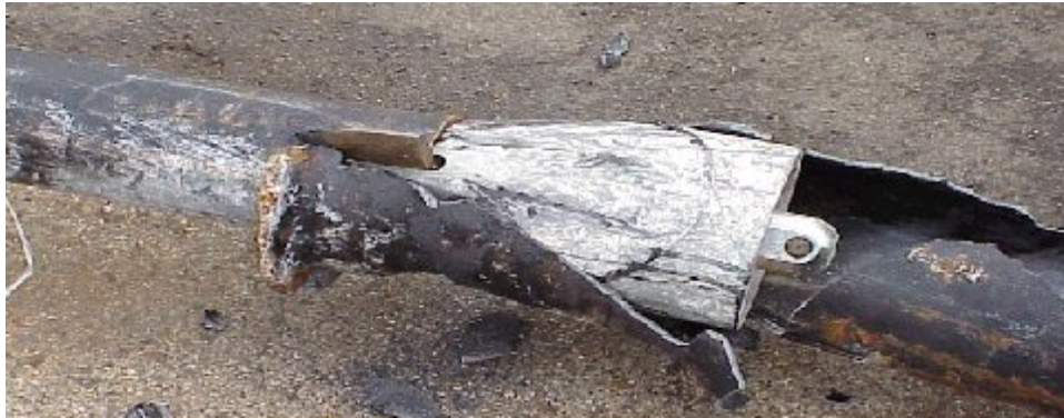
FIGURE 6.6: PIPE SPLITTING (Picture Courtesy of AUI INC)
