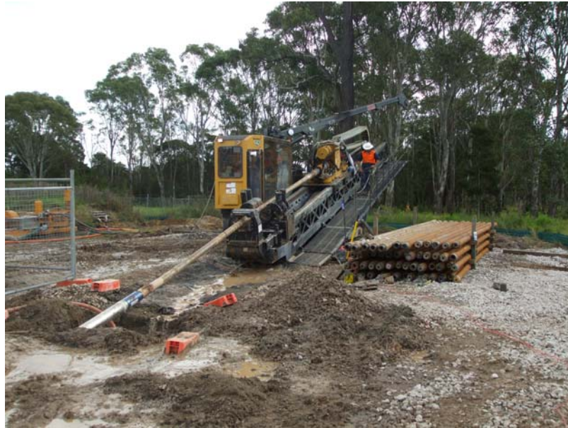
FIGURE 4.1: DRILL RIG (Picture Courtesy of UAE)
