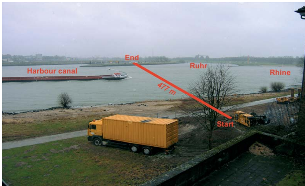
FIGURE 4.6: HDD UNDER CANAL
