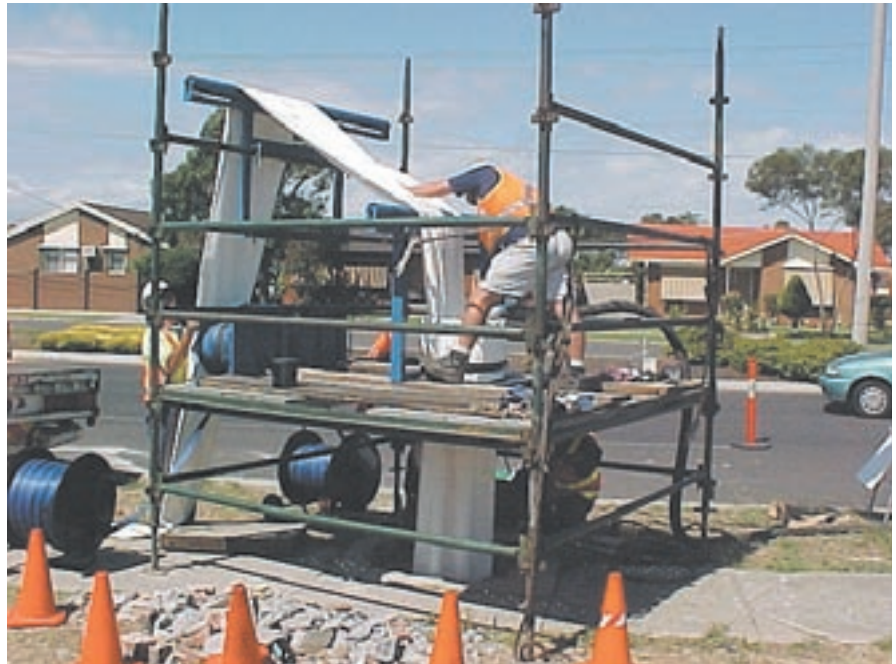
■ 180m length of liner installed in a 24 hr period
