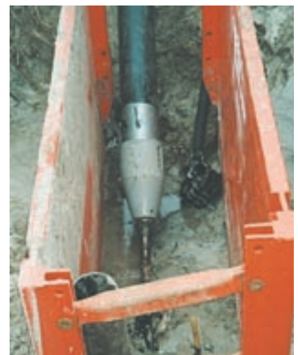
■ 420mm expander and the 350PE pipe being pulled into the pipe.
