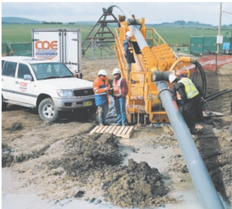
■ Coedrill 550 pipe pusher.
