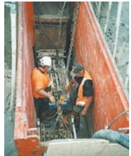
■ 800G ready to pull in pipe.
