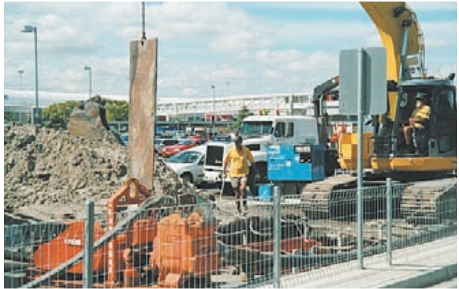
■ Brisbane Airport and the 800G in the dewatered excavation.
