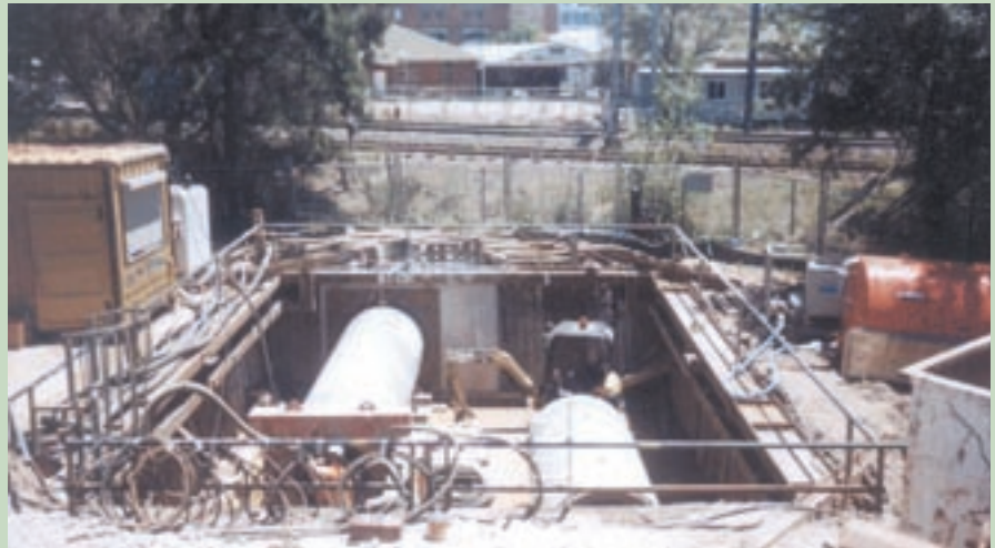
■ Railway line in background, control container in foreground.
