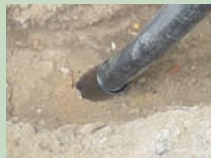
■ Removing the Quick Loks rods while pulling in the new PE pipe
