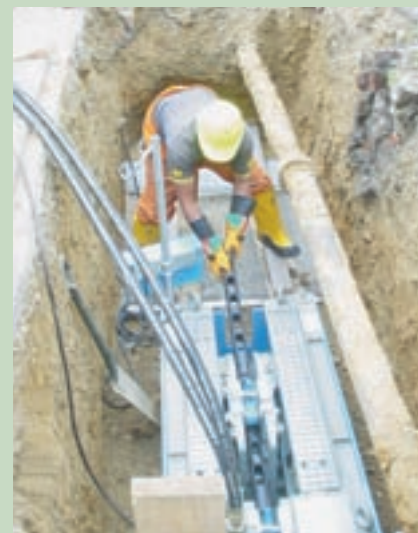
■ Removing the Quick Loks rods while pulling in the new PE pipe
