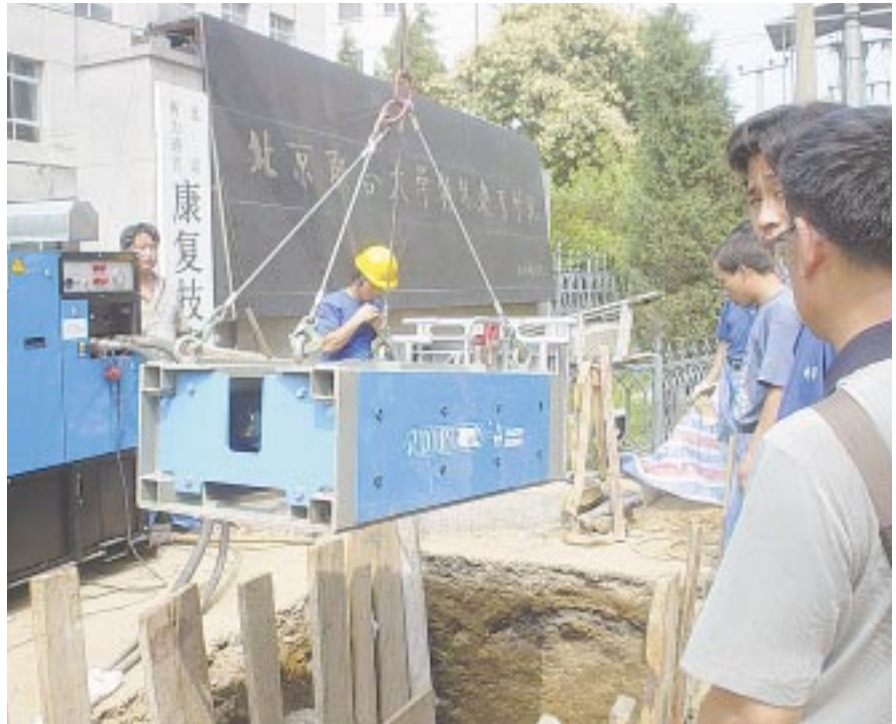
■ 800G machine and Power Pack ready for another Burst outside the Beijing Union University.
