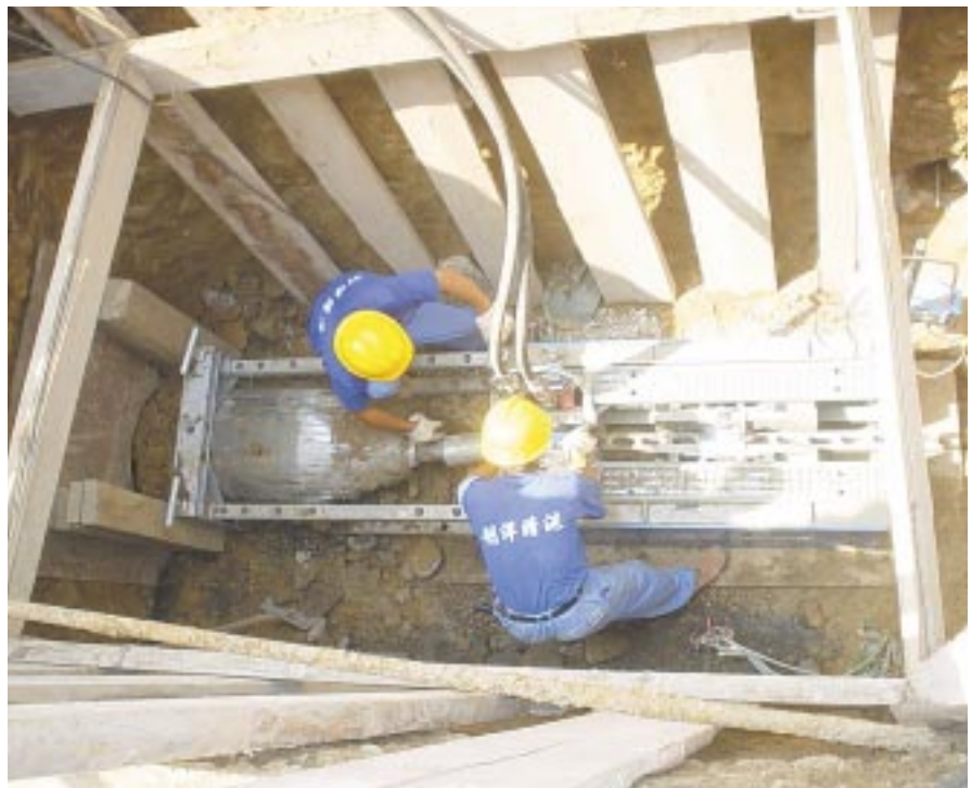
■ 800G machine and Power Pack ready for another Burst outside the Beijing Union University.
