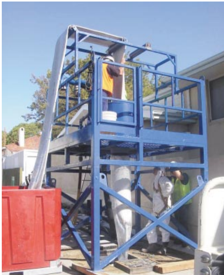
■ The pipe liner is installed using a specially built access platform.
